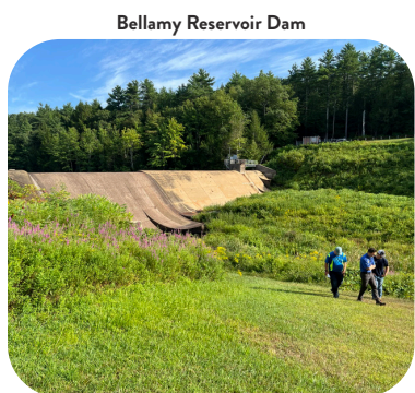
Bellamy Reservoir Dam
