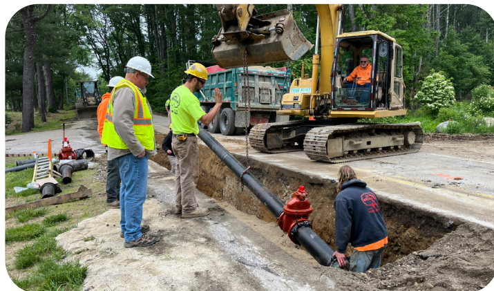
Installation of Little Bay Rd. water main.
