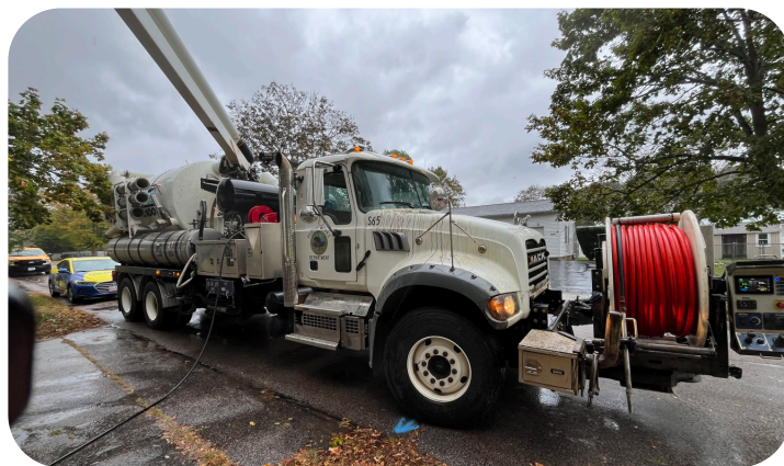
Service line identification efforts using a vacuum excavator.
