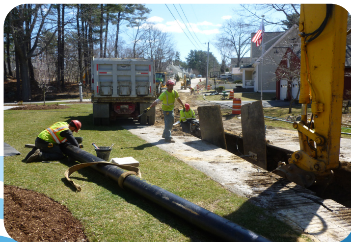
New Castle water main replacement.
