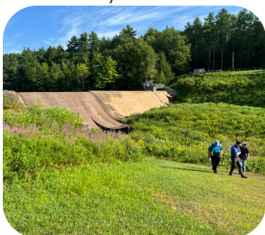
Bellamy Reservoir Dam
