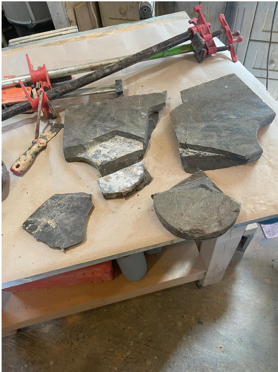
Part of a Hall headstone in front row – before applying epoxy.
