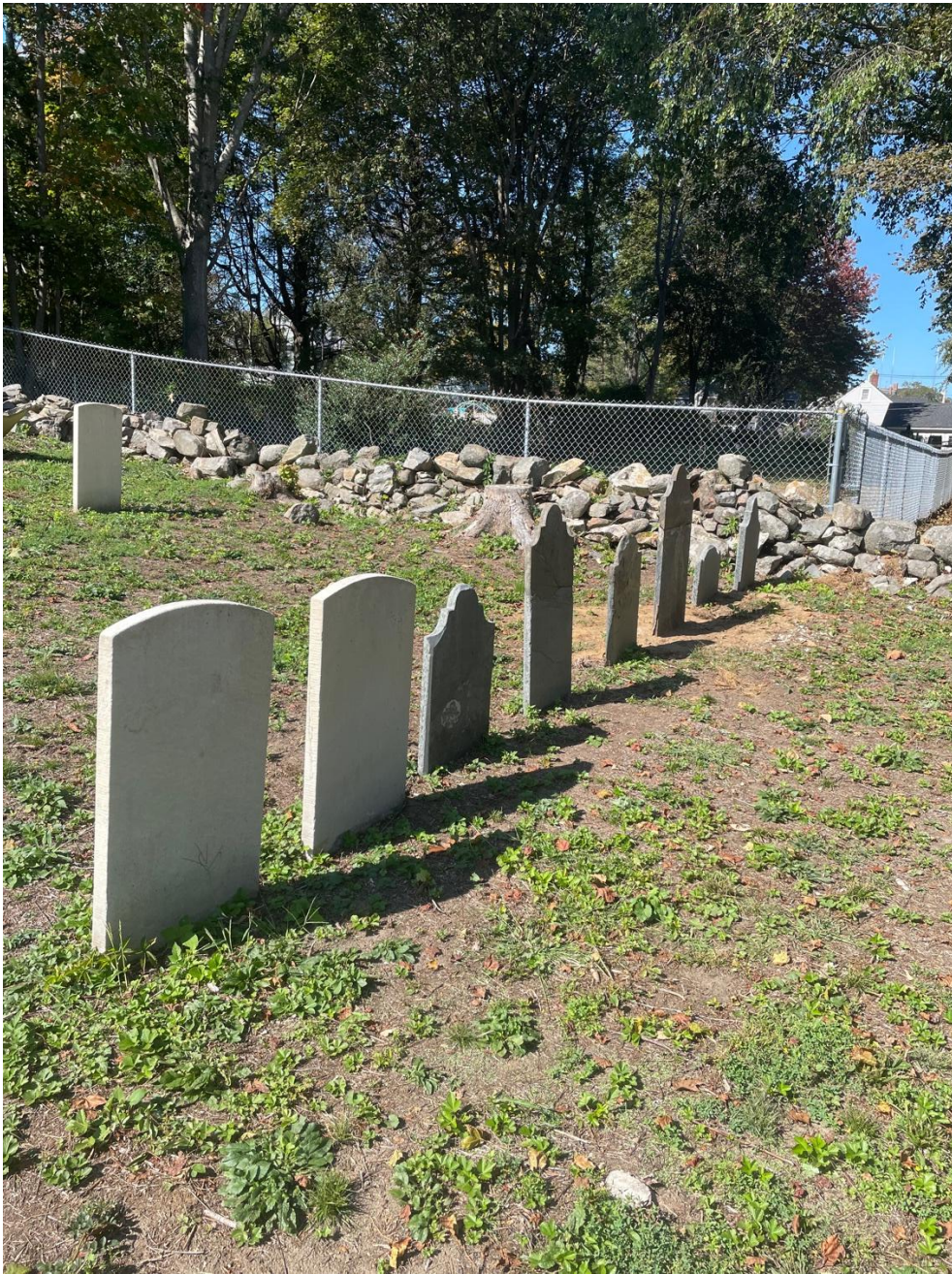
Front Row after resetting and epoxying. The headstone pieces (shown in previous picture) are part of the 4 th headstone from the left.
