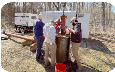
Portsmouth's Water Treatment Operators performing a pump test on Greenland's backup well.
