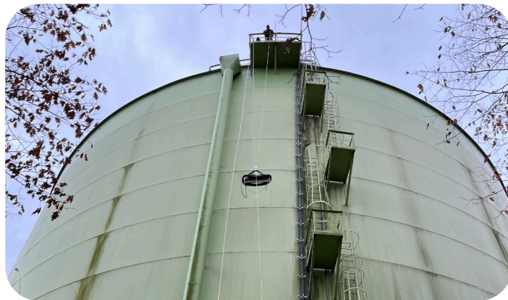
Installation of water mixing system at Lafayette Storage Tank.
