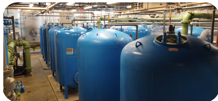
Resin vessels at the Grafton Road Water Treatment Facility.
