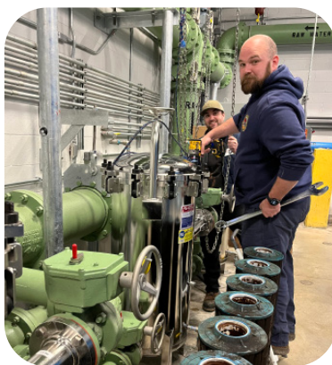
Pease Water Treatment Operators replacing cartridge filters.
