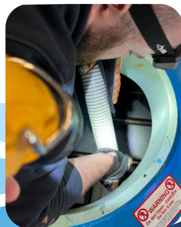
Loading of new ion-exchange resin media into existing vessels.
