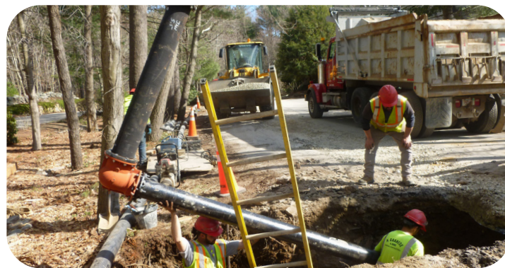
Hydrant installation on Spring Hill Rd. in New Castle
