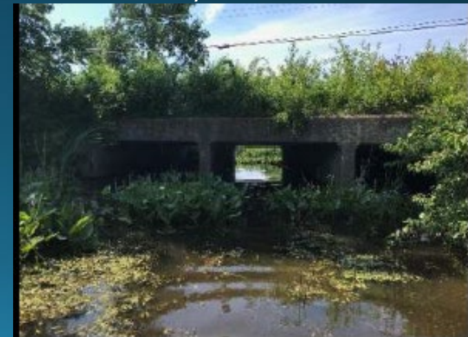
Coakley Road Culvert
