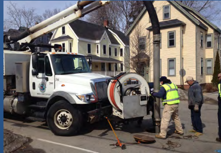
Catch Basin Cleaning - 322 Tons cleaned in 2018
