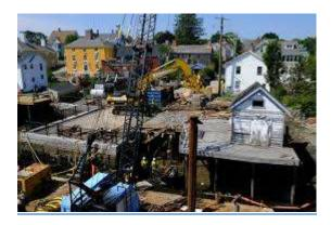
**95 MECHANIC STREET SEAWALL RECONSTRUCTION** – Dewatering and seawall demolition. Delivery of H-beams and other small materials later this week. For more information and to subscribe to email updates on the project, click here: <a href="https://tinyurl.com/w48zy332">https://tinyurl.com/w48zy332</a>
