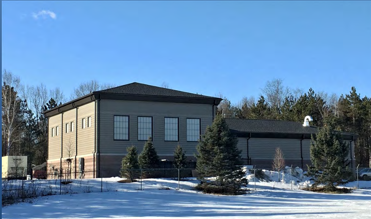
Water – Pease Water Treatment
