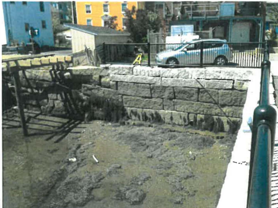
Photo 4: This photo shows the proposed location of the landing and gangway access to the proposed floating docks, taken from the point of the seawall bump out looking south, taken on 6-24-2019.
