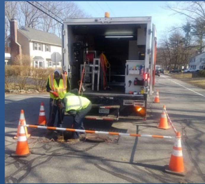
Pipe Inspections and Cleaning - 7,800 Feet in 2019
